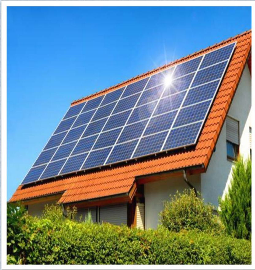
Solar Roof Top
